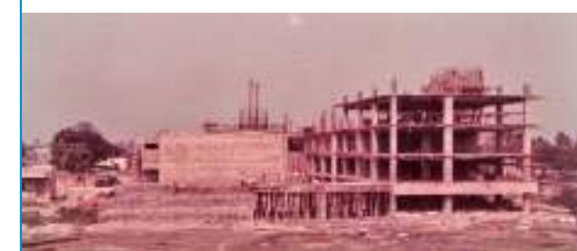
Madhusudan Manch Under Construction at Dhakuria
